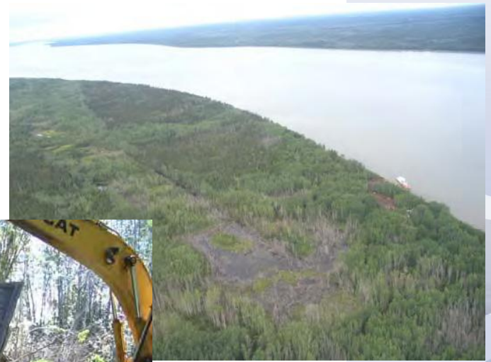
Aerial view of Axe Point during remediation
