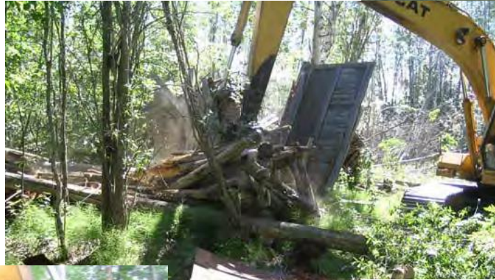
Demolition of Garage structure
