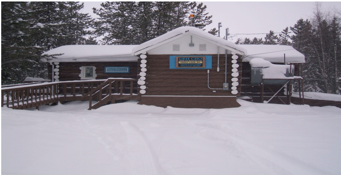
Dehcho Health and Social Services Authority facilities in Trout Lake.
